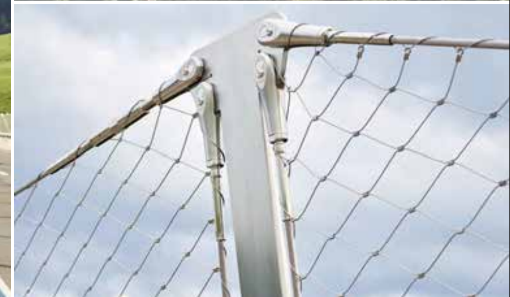
Hundwilertobelbrücke, Appenzell AR (CH)
